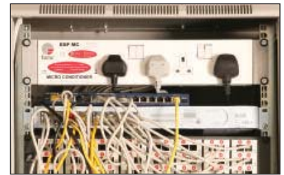
ESP MC installed within a network rack, protecting the externally-fed network switch
